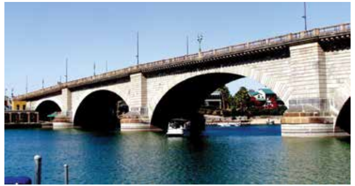
London Bridge in Lake Havasu City.
