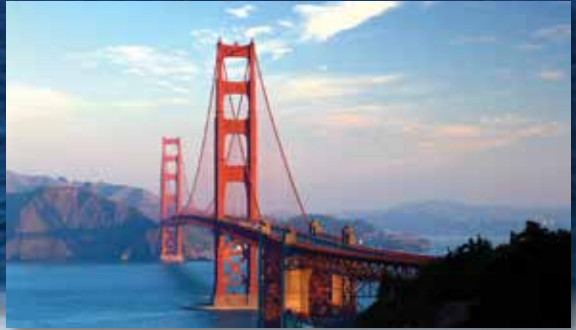
San Francisco's historic Golden Gate Bridge.
