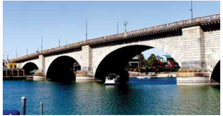
London Bridge in Lake Havasu City.
